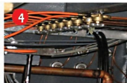
Isolation Valve - Reduce risk of malfunction and increase in safety usage - Easier parts replacement
